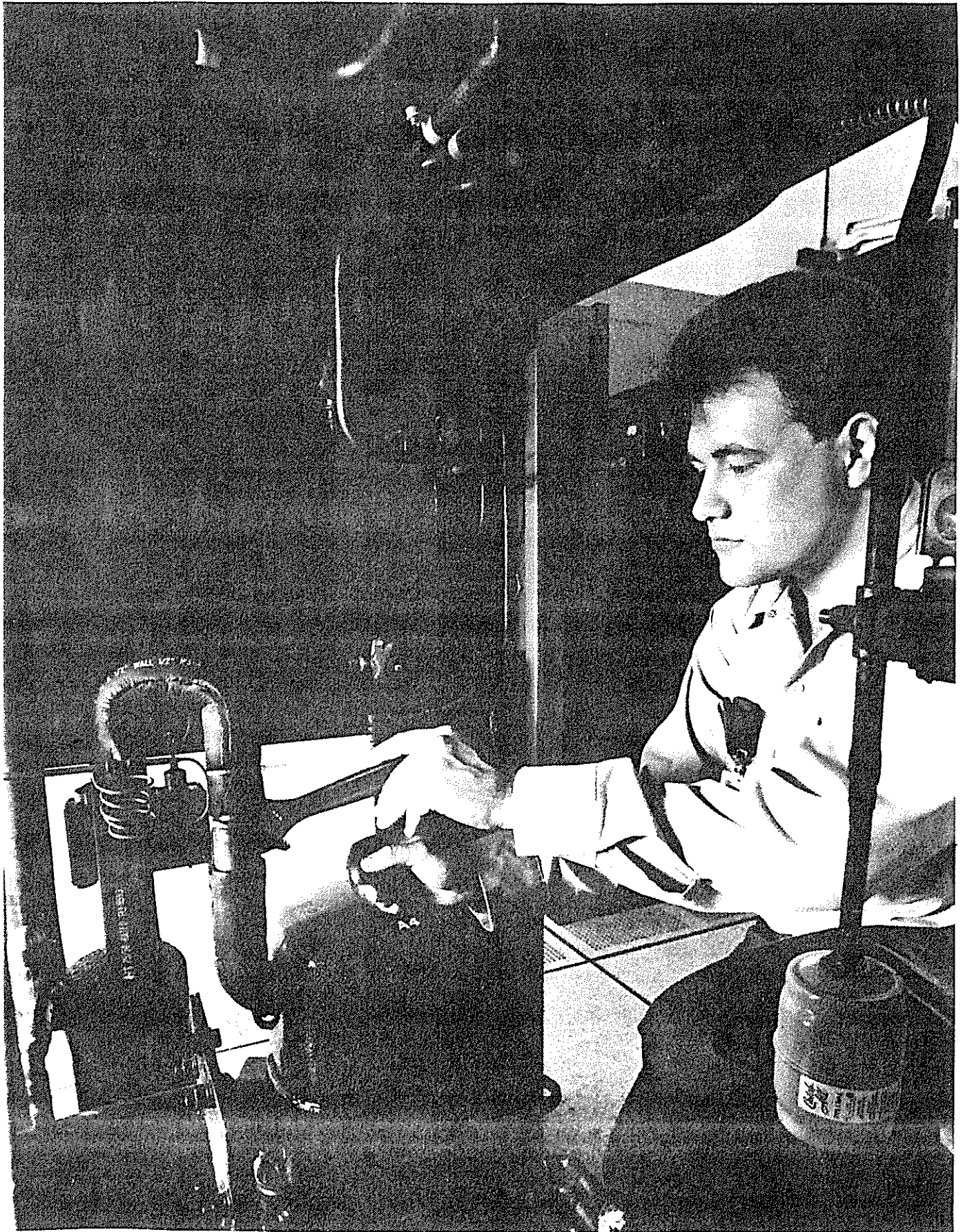
Air Conditioning and Refrigeration
